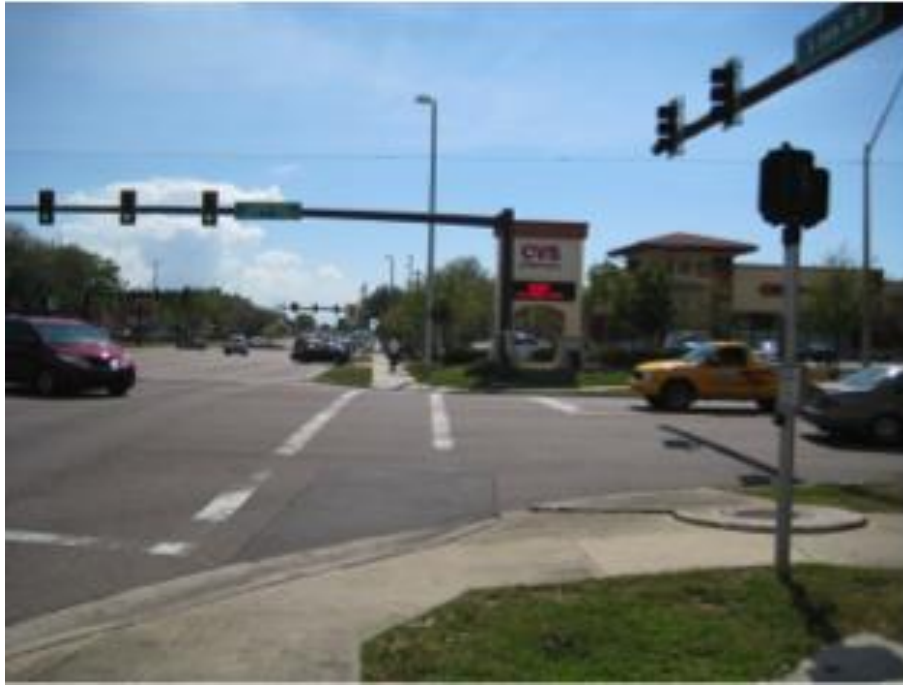
Figure 4 Brick paver crosswalk with white outline
